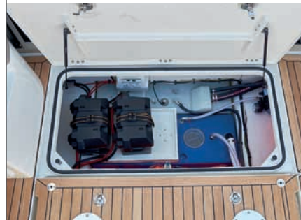
Storage below cockpit floor
